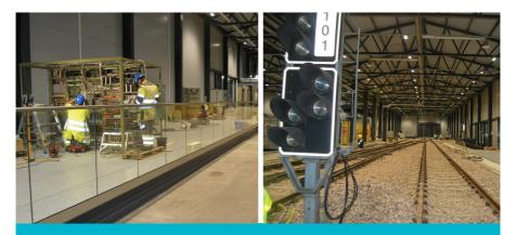
There is a rail connection from the facilities with signalling and interlocking systems to the outdoor track area with an electrified railway line for training purposes. The facilities have been equipped with two electrically operated turnouts, a so-called elastic turnout and a double slip. Turnouts can be controlled via the interlocking devices.
